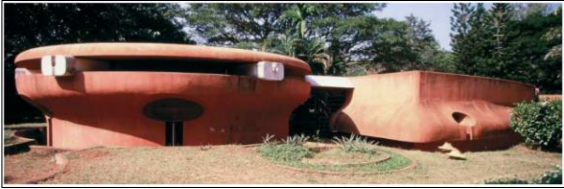
Figure 10 Roger Anger's Sanskrit School, Auroville, 1971. Here, free-flowing spaces held by free-flowing playful forms were realized while experimenting with ferrocement technology that permits almost any shape
