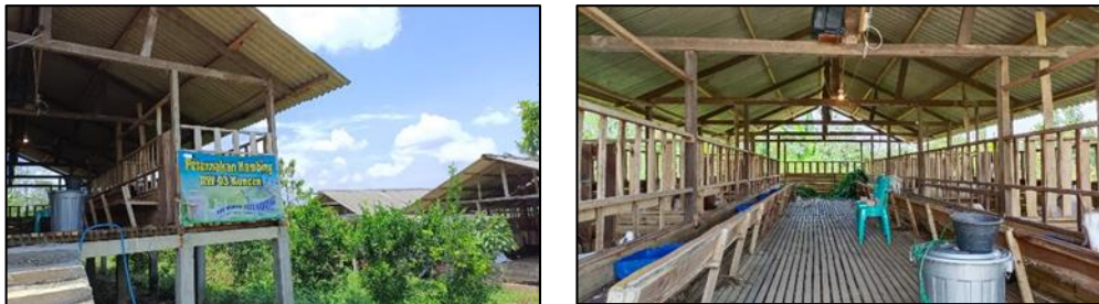
Figure 9 Outside and Inside Conditions of the Cage
